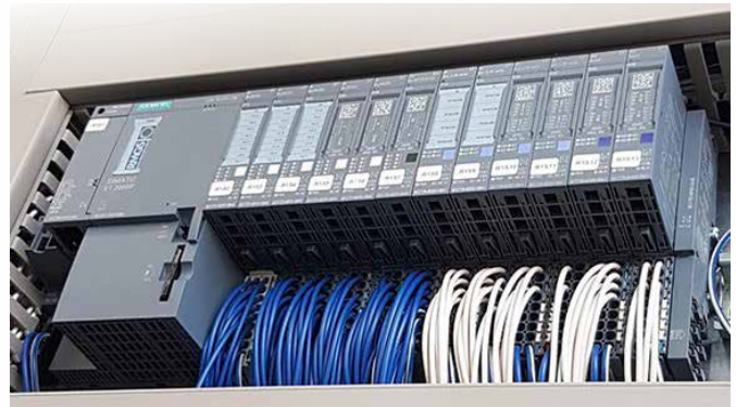
Beispiel: SCS 2010 by RMGS®, AS Hardware Simatic S7 1500, Bauform ET200SP
