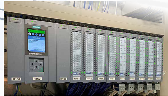
Beispiel: SCS 2500 by RMGS®, AS Hardware Simatic S7 1500, Bauform ET200MP
