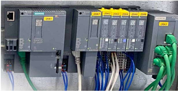
Beispiel: ECS 2020 by RMGS®, AS Hardware Simatic S7 1500, Bauform ET200SP
